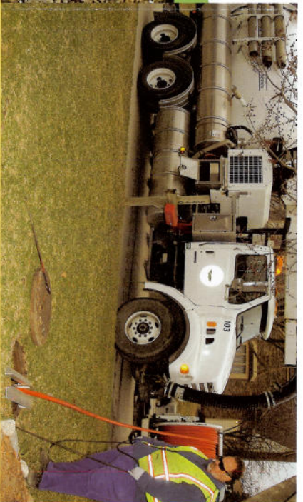
FOG build-up in sewer pipes (shown below) is costly to clean requiring local public works staff to go to the site and remove the blockage (shown above).
